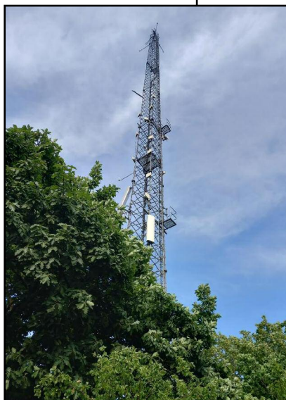
The radio mast on Horniman Drive
